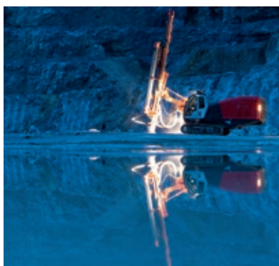
The DI550 surface down-the-hole drill rig at work.
